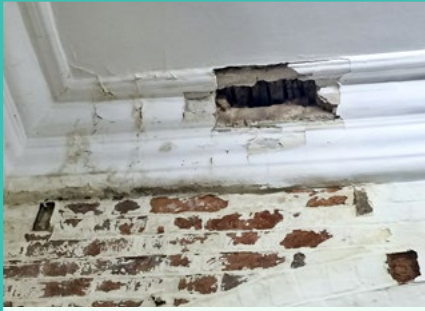
◀ 簷口和牆壁因為屋頂長期滲水而被損壞。 Cornice and wall damaged by long-standing water seepage from the roof.
